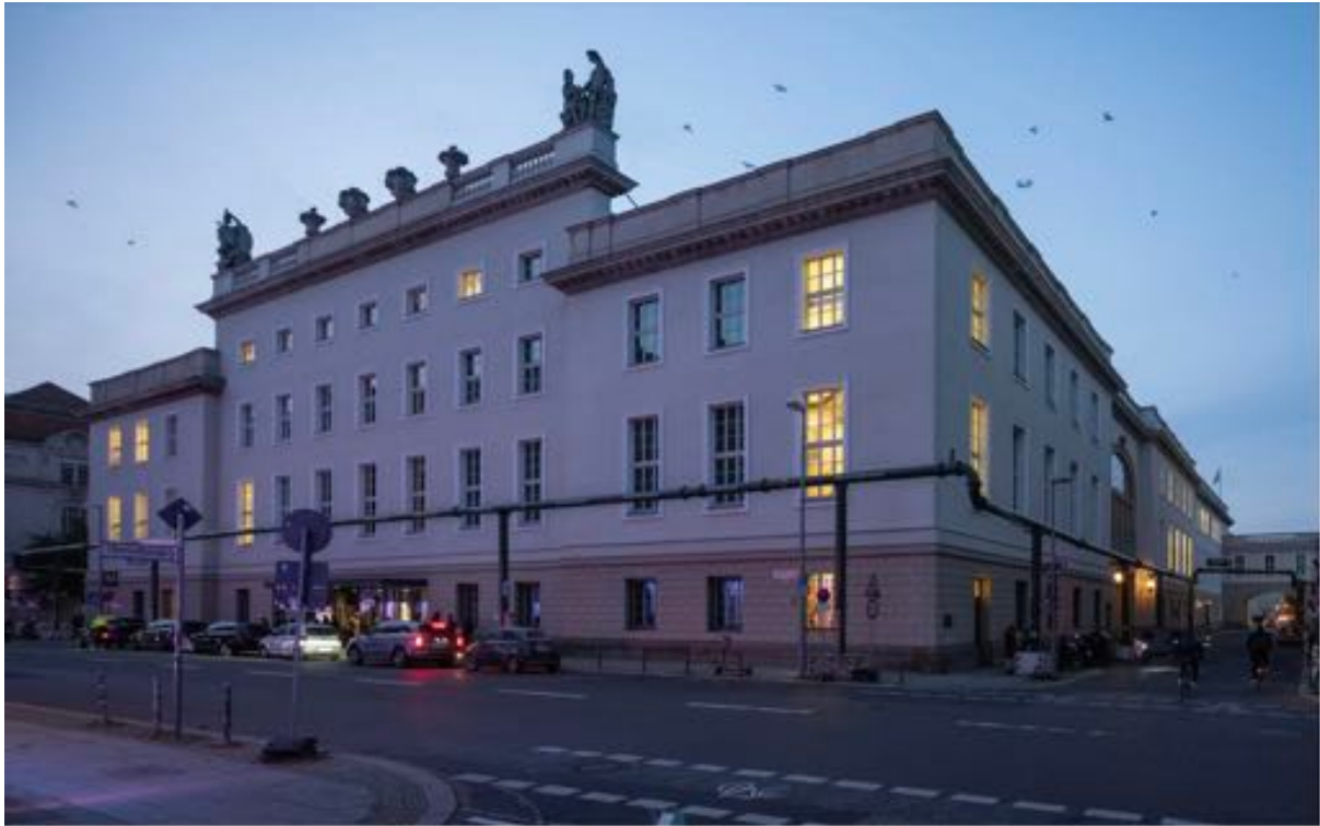
The academy was built in an old opera warehouse in the heart of Berlin whose exterior was preserved while its interior was gutted and rebuilt. Andreas Meichsner for The New York Times
